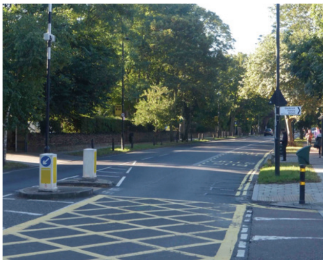
Figure 24: Median islands placed just ahead of bus stops help departing buses rejoin the traffic stream without delay and also help pedestrians cross to reach the bus stop (King's Avenue, London). (Photo: Tim Pharoah, 2016)
