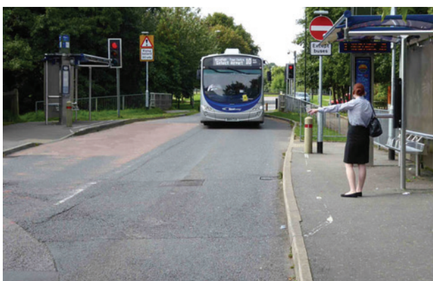
Figure 27: Bus gate enforced with rising bollards, providing preferential routing for buses (Crawley, West Sussex). (Photo: Tim Pharoah, 2017)
