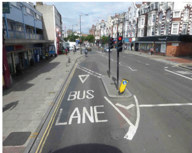
Figure 25: Bus lane with separate traffic signal provides priority for buses to re-enter the traffic stream, with light control (Walworth Road, London) (Photo: Tim Pharoah, 2017)
