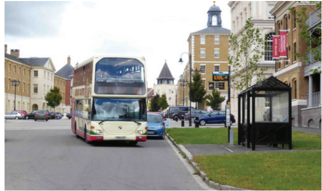
Figure 38: Parking in advance of the stop limits ability to bring bus adjacent to the kerb. A bus boarder would resolve the problem. (Photo: Tim Pharoah, 2017)
